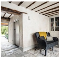
Use of Lime plaster on the wall and wooden beams on ceiling
