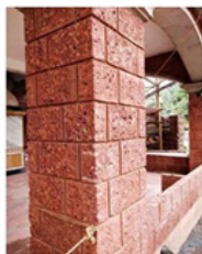
Laterite stone used for walls and columns
