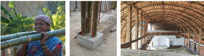
Use of Bamboo in columns construction of columns, beams and arches
