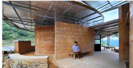
Rammed earth construction of the wall
