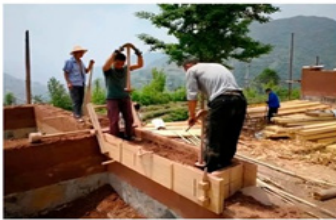
Rammed earth construction of the wall
